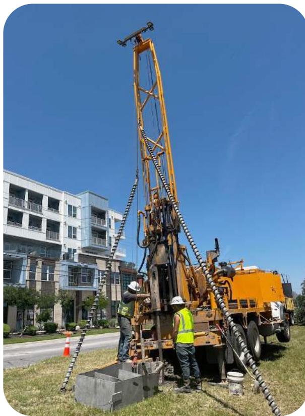
ATP conducting preconstruction activities.
