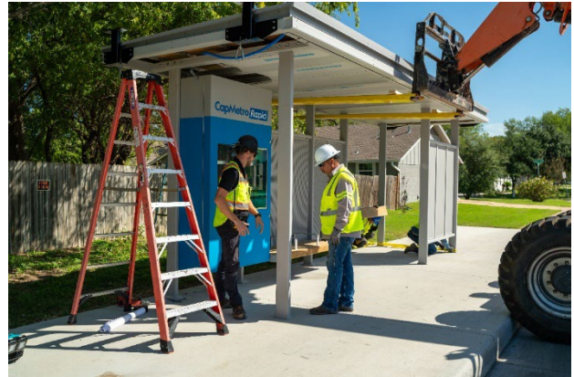
CapMetro Rapid Shelter
