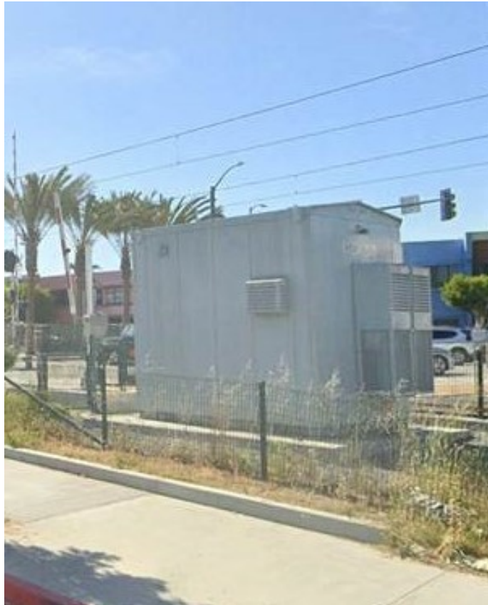
Example of a Train Control Bungalow (LA Metro, Los Angeles, California)
